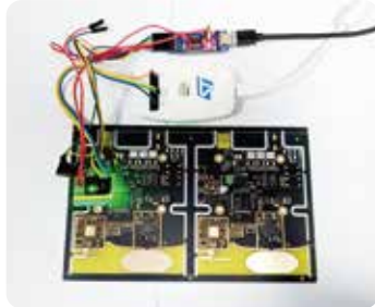
Test of Semi-automatic Control Function
